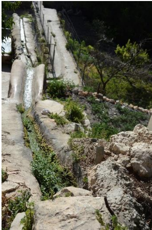
Figure 5-2: A portion of the water-conveyance system
